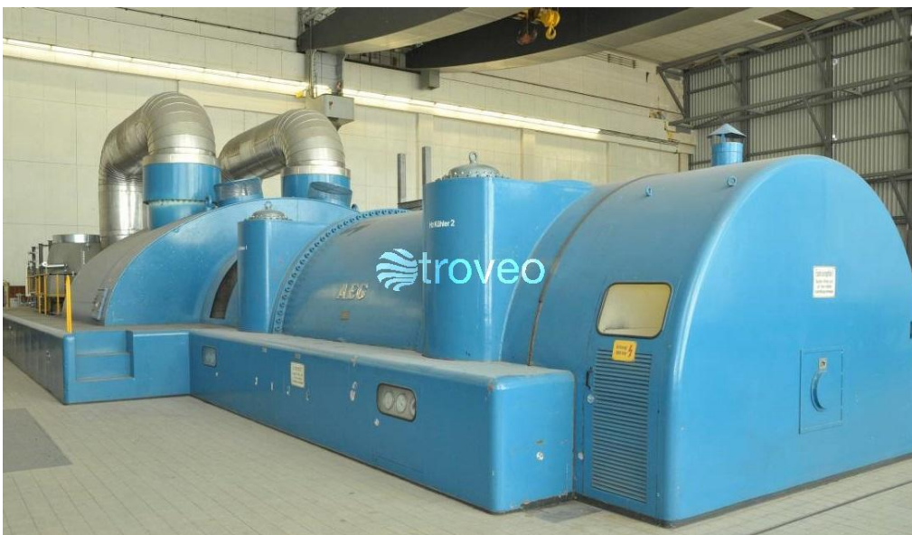
turbine generator set
